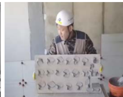
Art wall epoxy spot bonding
