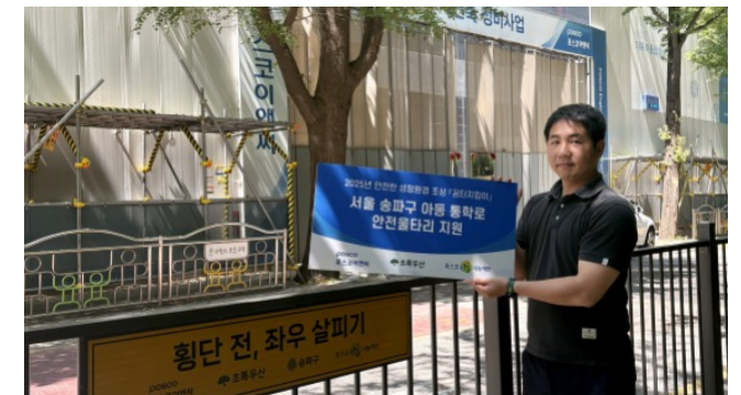
'Dream Space Guardian' Safety Fence Repair
