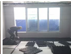
Anwoollim inter-floor sound insulation structure
