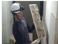
Tile: bathroom renovation spot bonding
